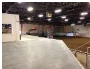
New mezzanine & lights at Calnash Ag Centre
